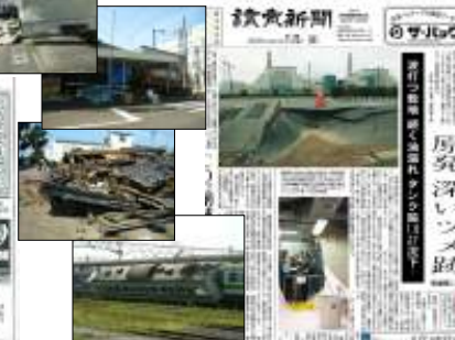
"Heavy damages remains in the nuclear power plant" Yomiuri , July 22, 2007
